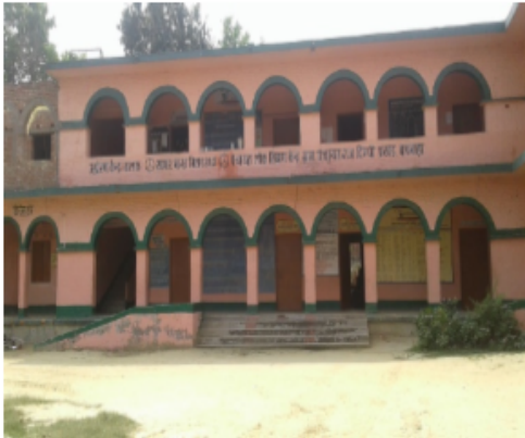
Polling Station Building Front View
