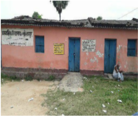
Polling Station Front View
