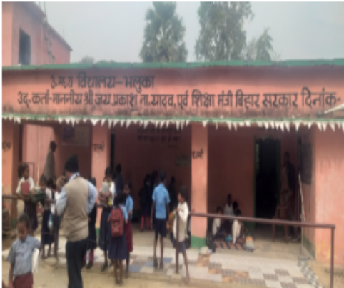
Polling Station Front View
