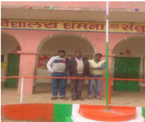
Polling Station Front View
