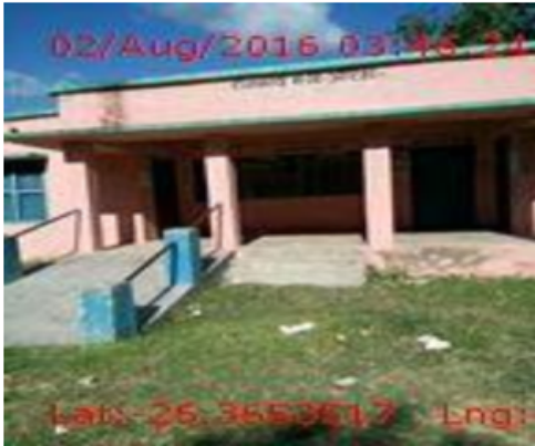
Polling Station Building Front View
