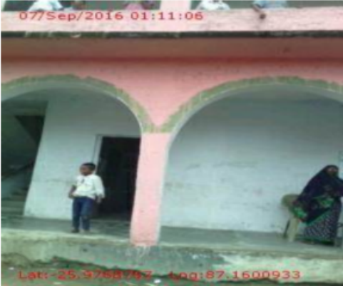
Polling Station Building Front View
