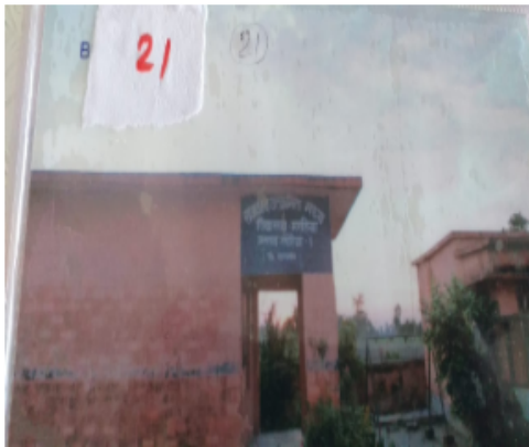
Polling Station Building Front View
