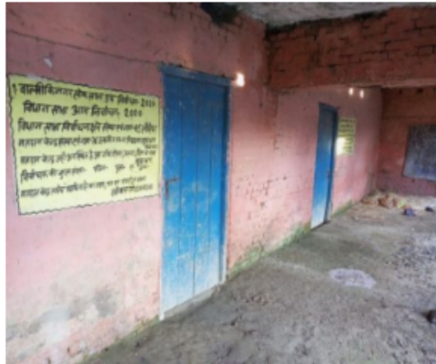
Polling Station Building Front View
