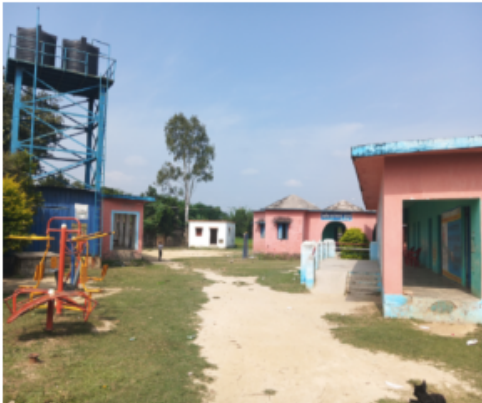
Polling Station Front View
