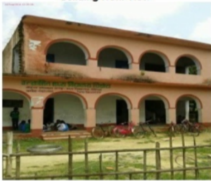
Building Front View
