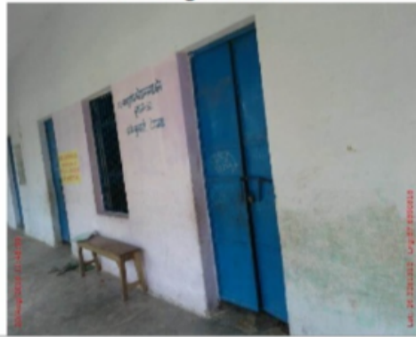
Building Front View
