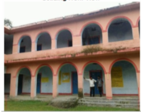
Building Front View
