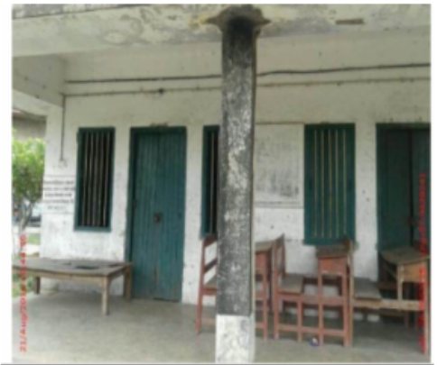
Polling Station Front View
