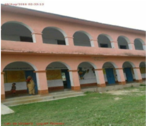
Polling Station Front View
