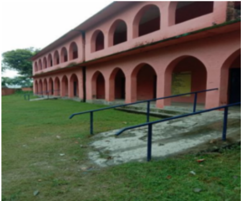
Polling Station Front View
