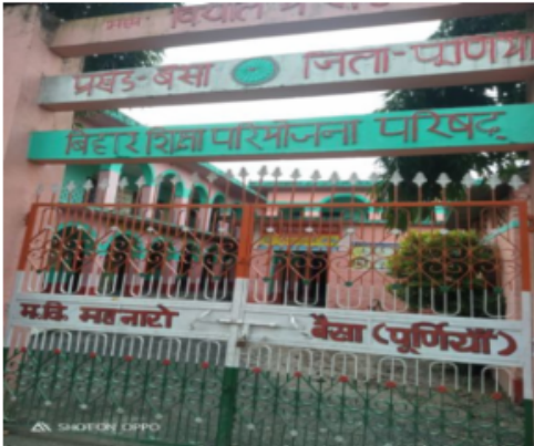
Polling Station Front View
