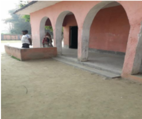
Polling Station Building Front View
