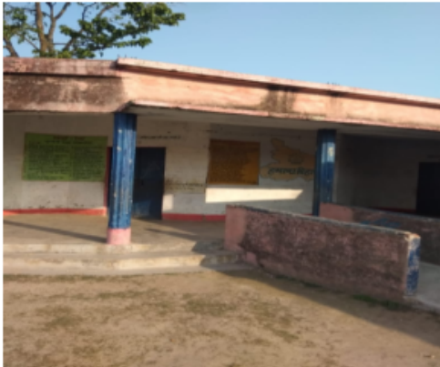
Polling Station Building Front View
