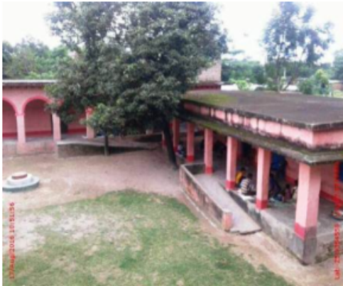
Polling Station Building Front View
