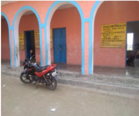
Polling Station Building Front View
