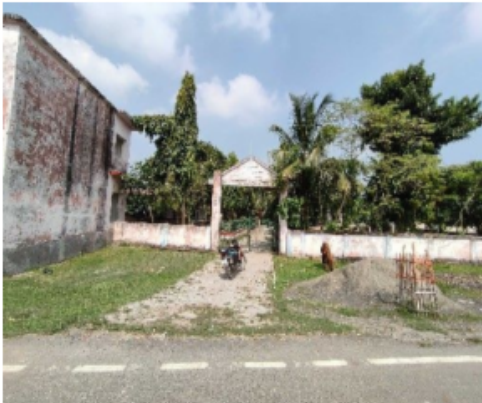
Polling Station Front View
