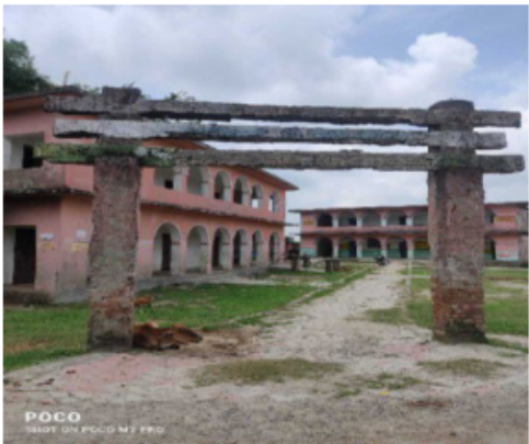
Polling Station Front View
