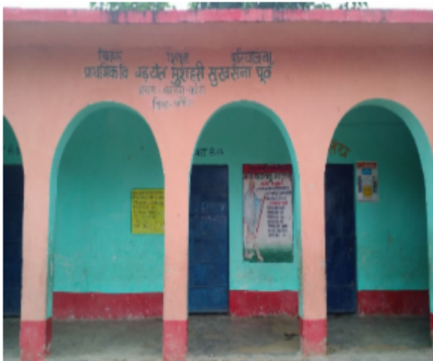
Polling Station Building Front View
