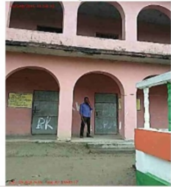
Building Front View
