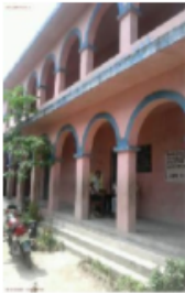
Polling Station Front View
