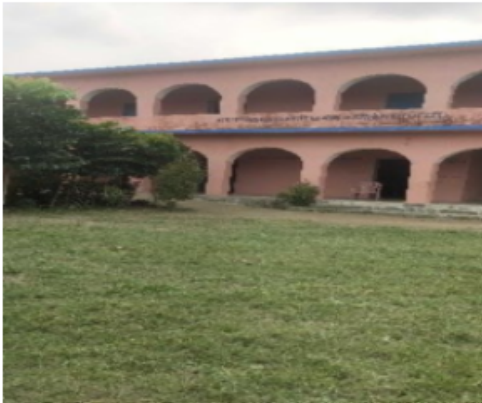
Polling Station Front View
