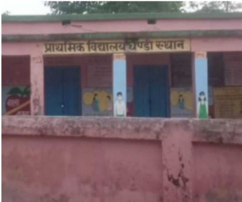
Polling Station Front View
