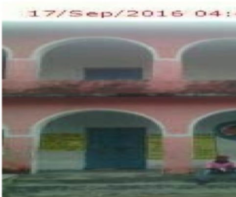
Polling Station Front View
