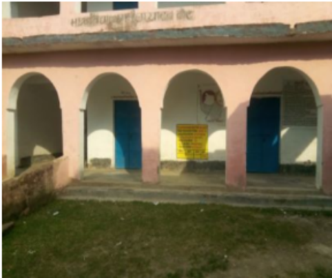
Polling Station Front View
