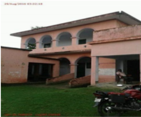
Polling Station Front View
