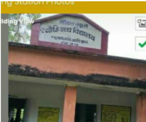
Polling Station Front View
