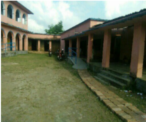
Polling Station Building Front View
