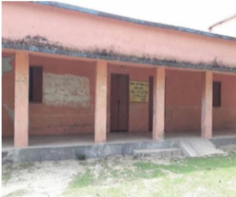
Polling Station Building Front View
