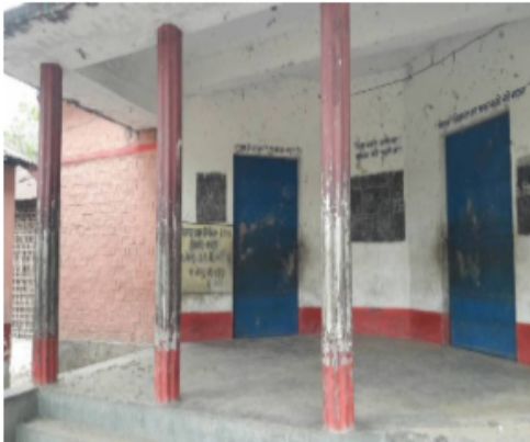
Polling Station Building Front View
