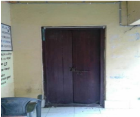
Polling Station Building Front View
