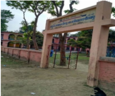
Polling Station Building Front View
