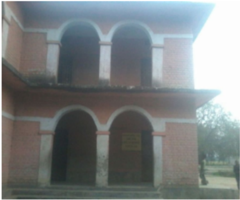
Polling Station Building Front View
