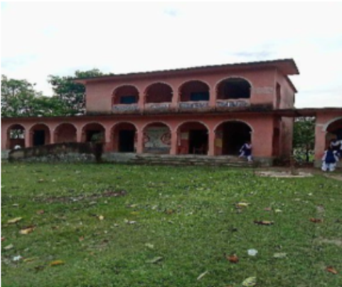
Polling Station Building Front View
