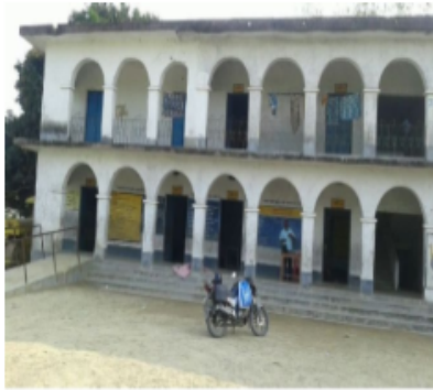
Polling Station Building Front View
