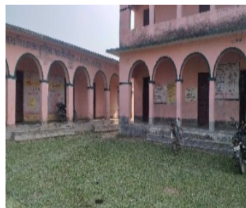
Polling Station Front View
