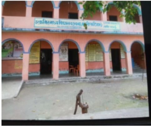
Polling Station Front View
