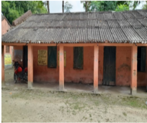
Polling Station Front View
