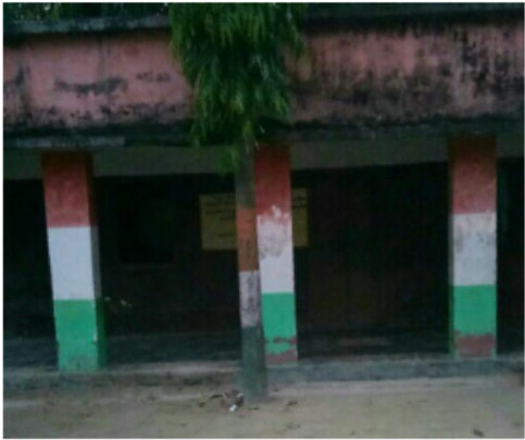
Polling Station Front View
