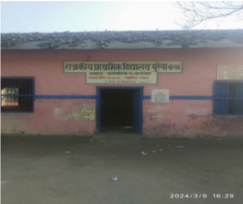
Polling Station Front View
