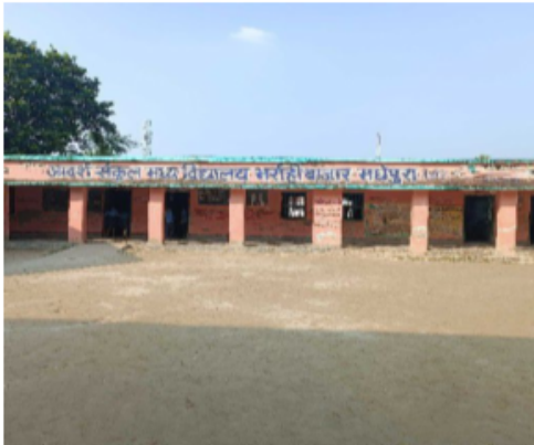
Polling Station Building Front View
