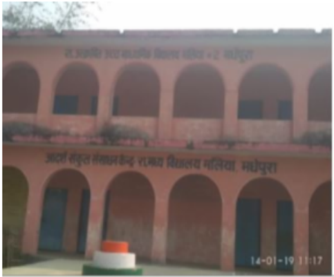
Polling Station Building Front View
