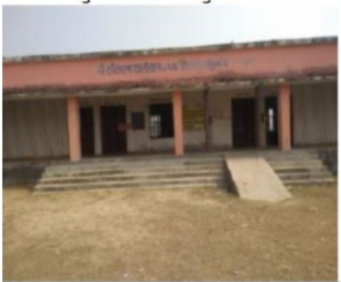
Polling Station Building Front View
