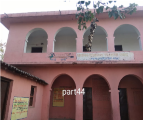
Polling Station Building Front View
