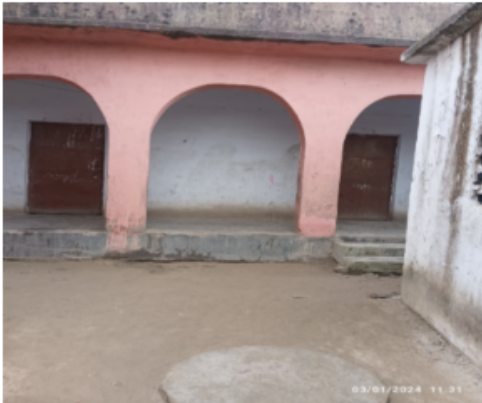
Polling Station Front View
