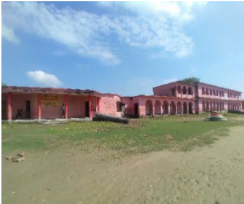
Polling Station Front View
